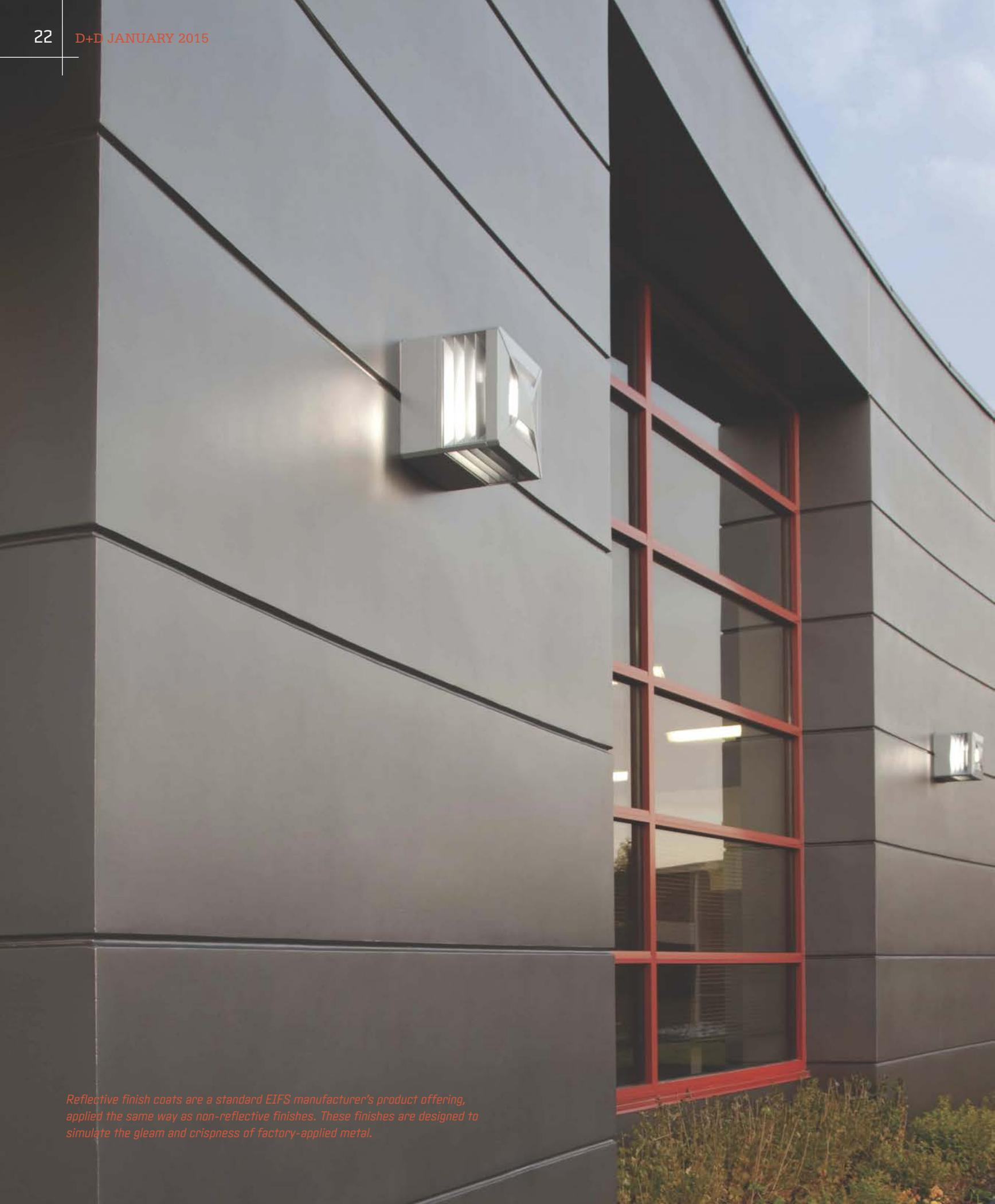
*Reflective finish coats are a standard EIFS manufacturer's product offering, applied the same way as non-reflective finishes. These finishes are designed to simulate the gleam and crispness of factory-applied metal.*
